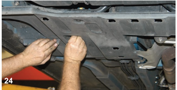
The plastic panel was installed using the fasteners that were carefully removed. Here one is being popped in place.
