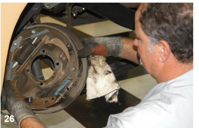
After the axle was removed the backing plate could be removed from the car.
